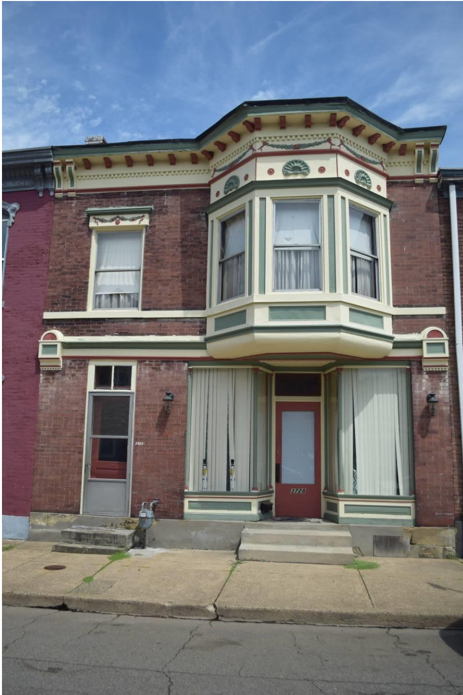
Photo 24. Storefront with residence at upper story, 3728 Eoff Street, looking northwest. (R#226)
