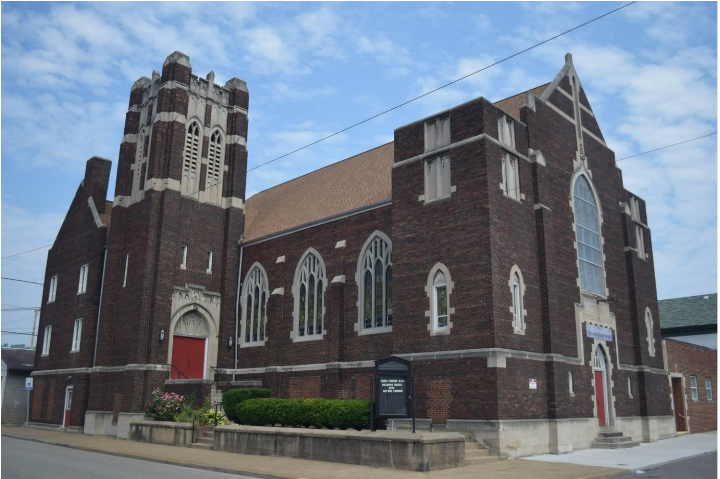
Photo 17. St. Paul's Evangelical Protestant Church, 3741 Wood Street, looking northwest. (R#274)
