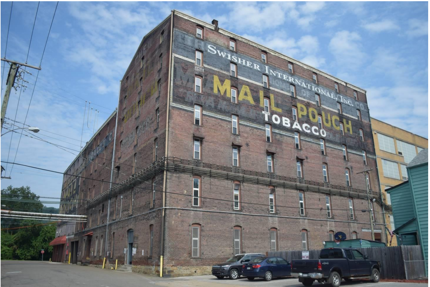
Photo 9. Bloch Brothers Tobacco, 3900 Water Street, looking northwest. (R#277 left, R#276 right)
