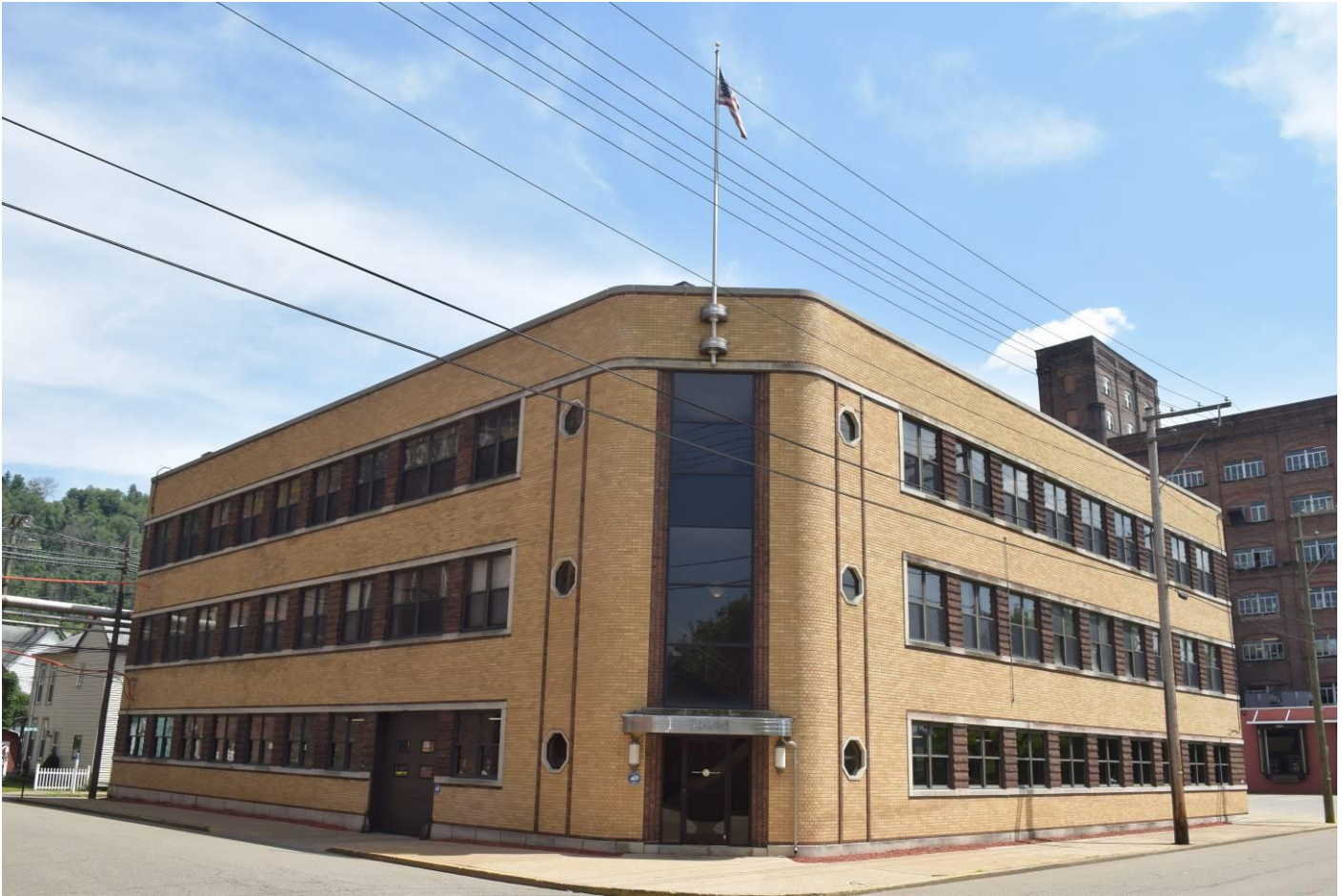
Photo 12. Bloch Brothers Tobacco, Office, 4000 Water Street, looking southeast. (R#279)
