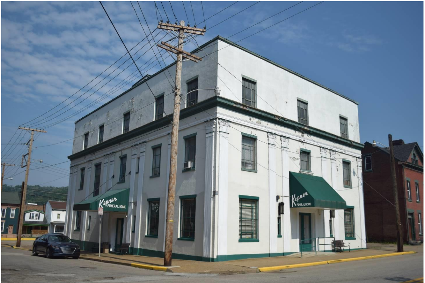
Photo 22. Kepner Funeral Home (formerly Handlan & Ratcliff), 3545-45 Jacob Street, looking northwest. (R#156)
