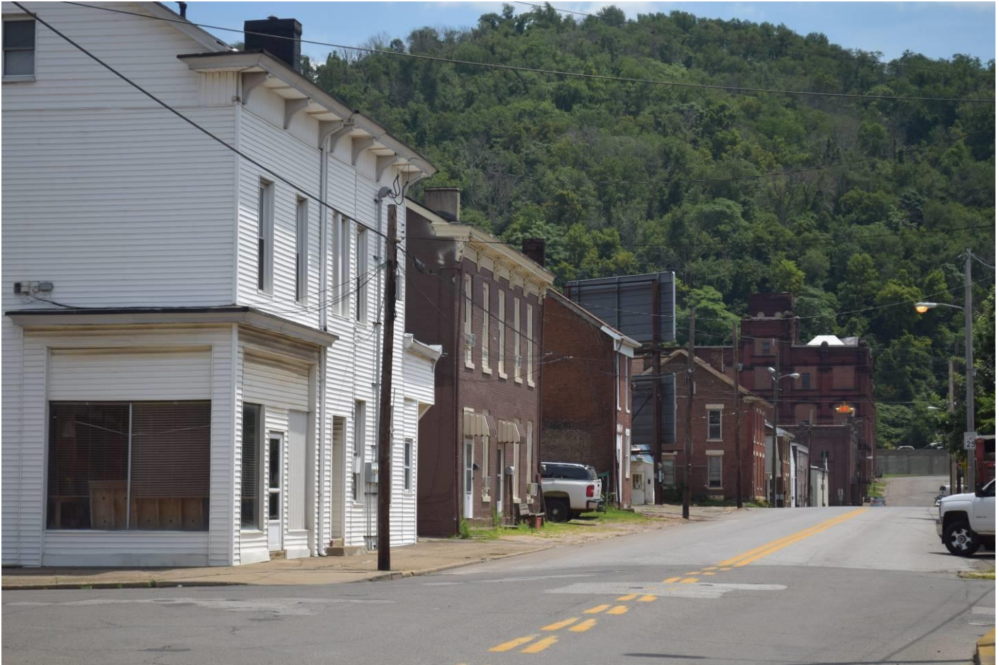
Photo 28. Streetscape, 33 rd Street, north side, from Eoff Street, looking east.
