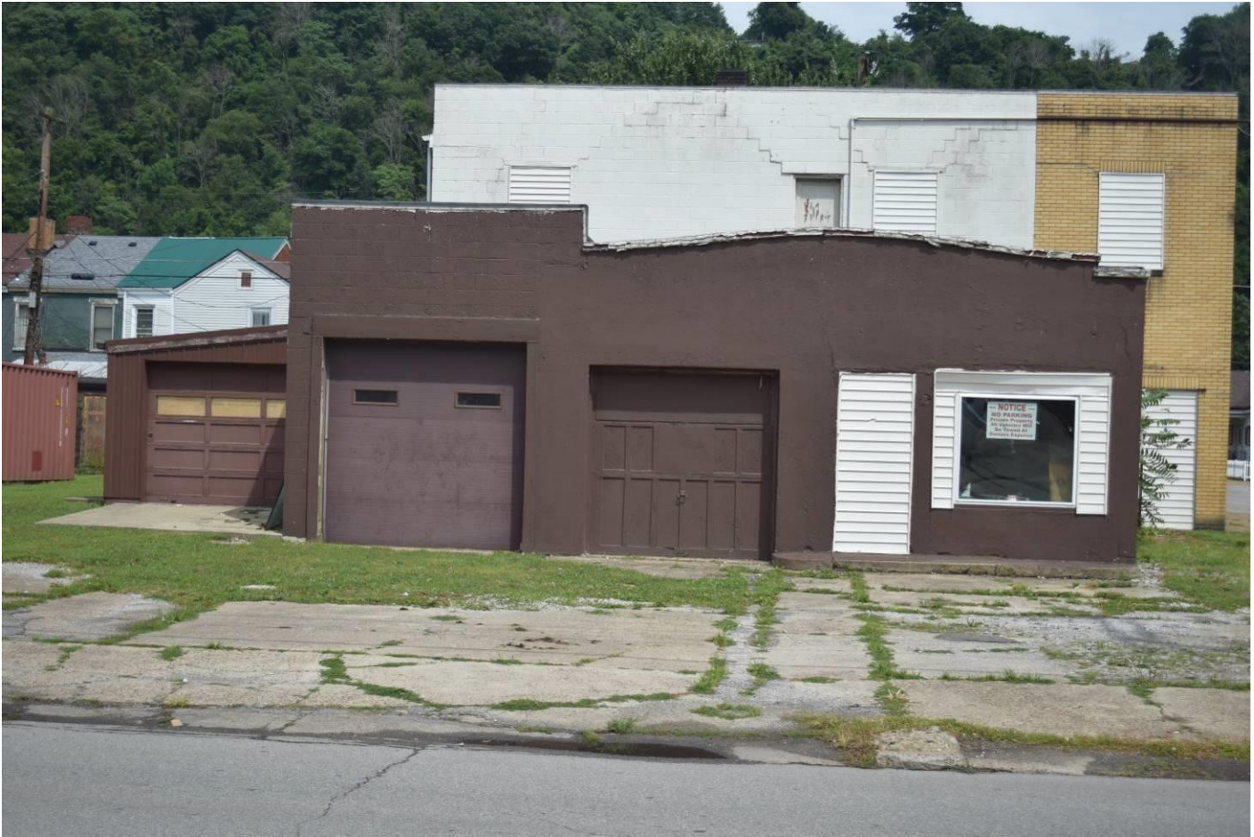
Photo 25. McLure's Service Station, 3942 Jacob Street, looking east. (R#310)
