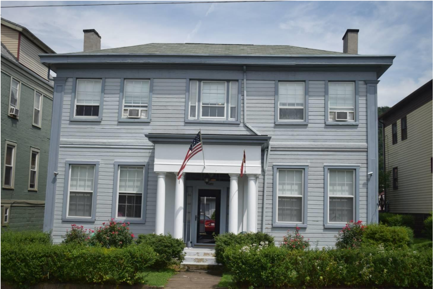
Photo 46. Greek Revival house, 3724 Chapline Street, oldest building in the district (1841), looking west. (R#179)
