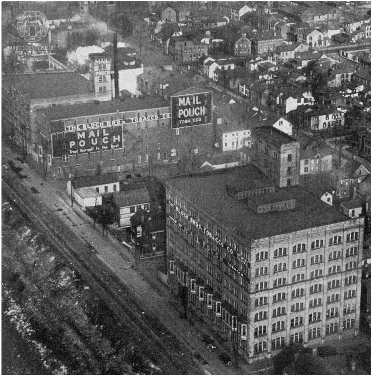
Historic Image 1. Aerial Photo, Bloch Bros. Tobacco, Water Street looking north, 1931. (Ohio County Public Library, Wheeling, WV)
