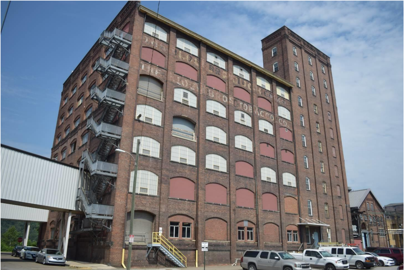
Photo 13. Bloch Brothers Tobacco, 4050 Water Street, looking northwest. (R#281 left, R#282 right)
