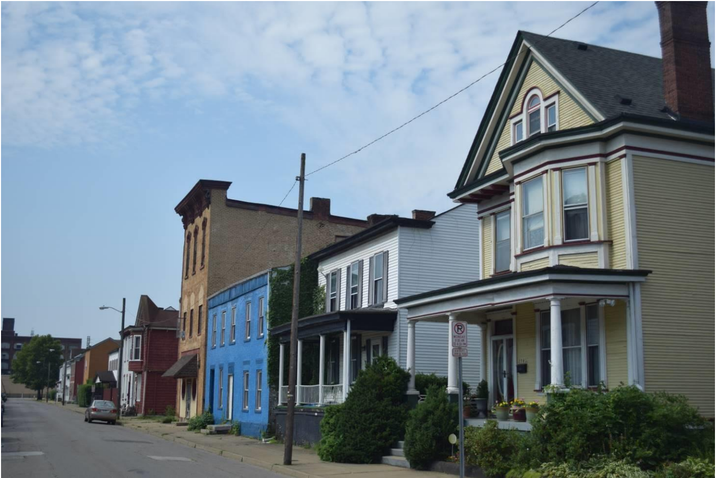
Photo 34. Streetscape, northern end of 3700 block of Eoff Street, west side, looking south.
