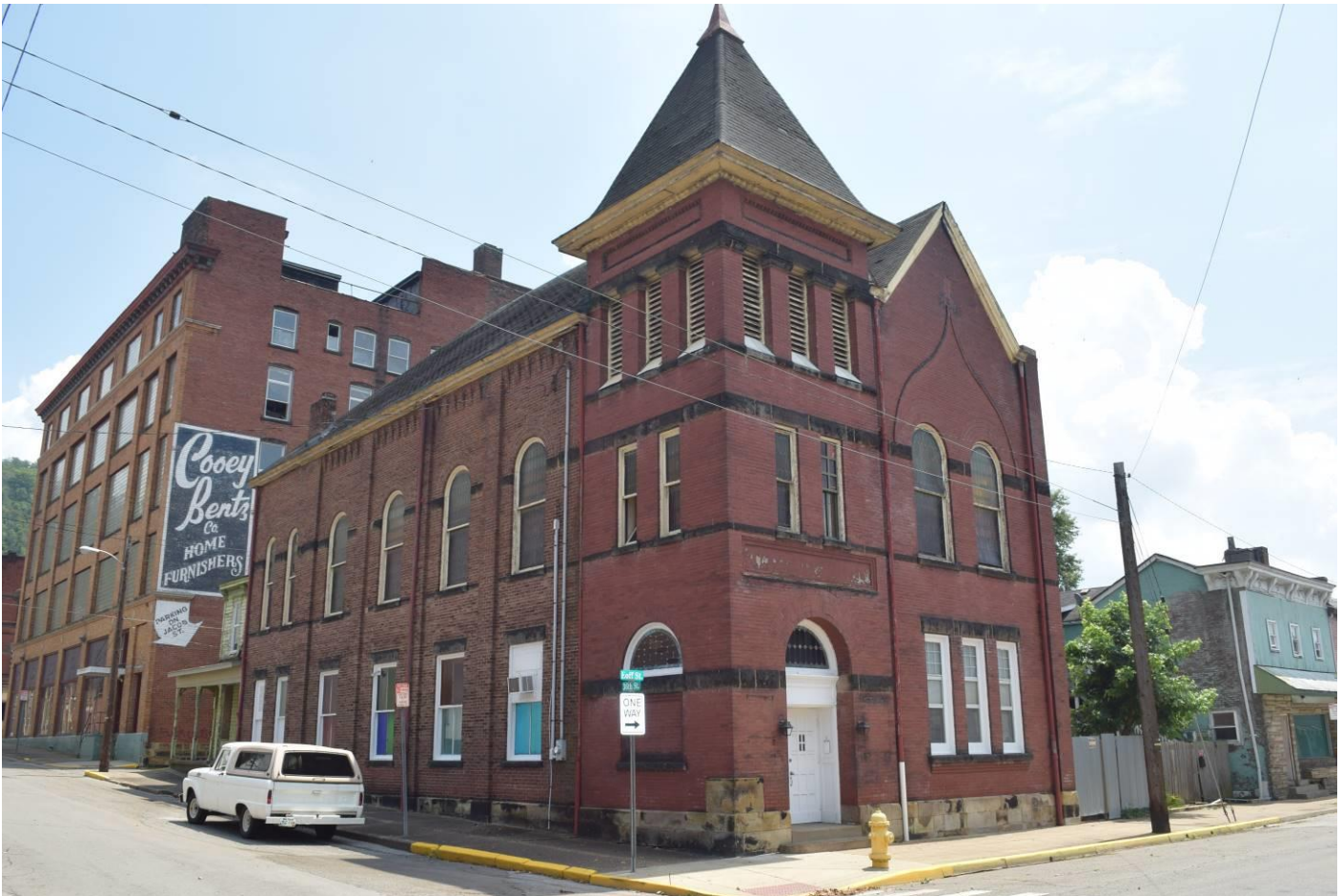
Photo 16. St. Stephen's German Reformed Church, 3600 Eoff Street, looking southeast. (R#133)
