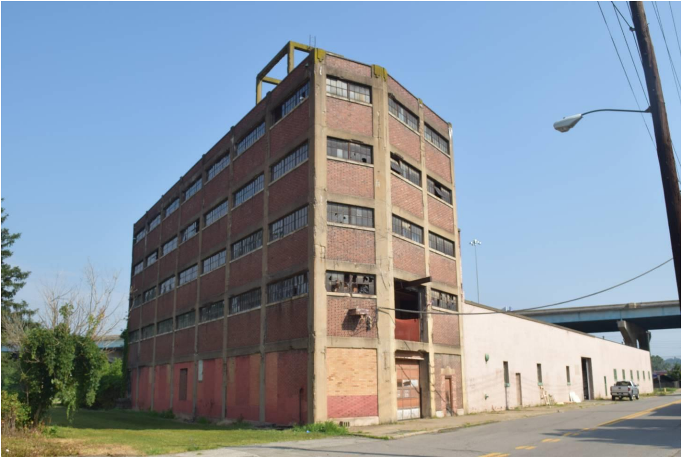
Photo 1. Wheeling Tile Plant 1, 3100 Chapline Street, looking northwest. (R#1)
