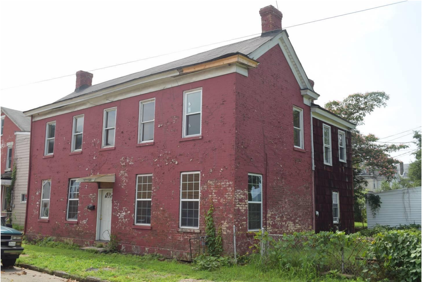
Photo 39. I-house, 6 38 th Street, looking southeast. (R#199)
