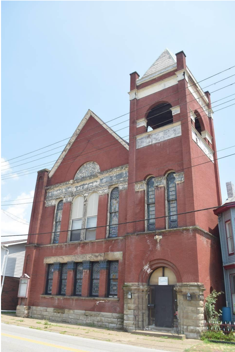
Photo 19. Third Presbyterian Church, 3806 Jacob Street, looking northeast. (R#265)
