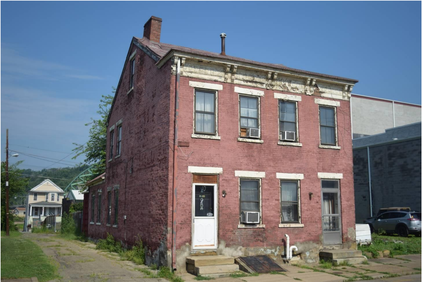
Photo 42. Italianate double house, 3317 Eoff Street, looking west. (R#71-72)
