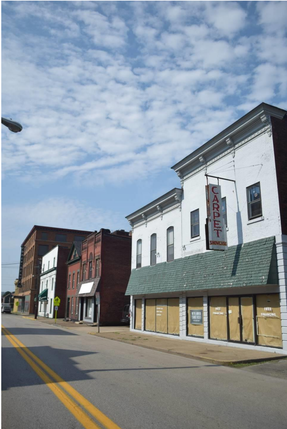
Photo 29. Streetscape, southern end of 3500 block of Jacob Street, west side, looking south
