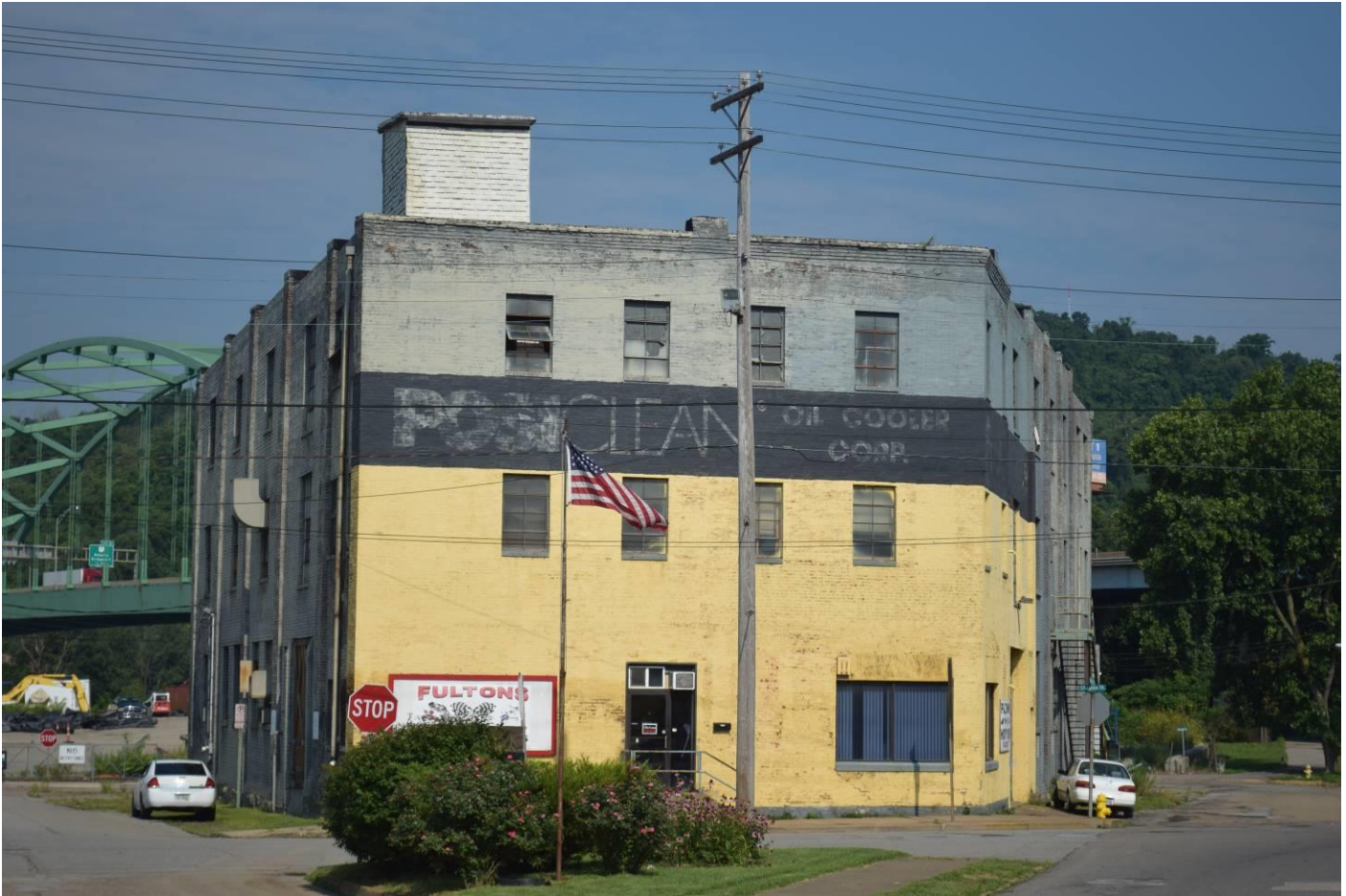
Photo 27. W.W. Wood Planing Mill, 3301 Chapline Street, looking west. (R#58)
