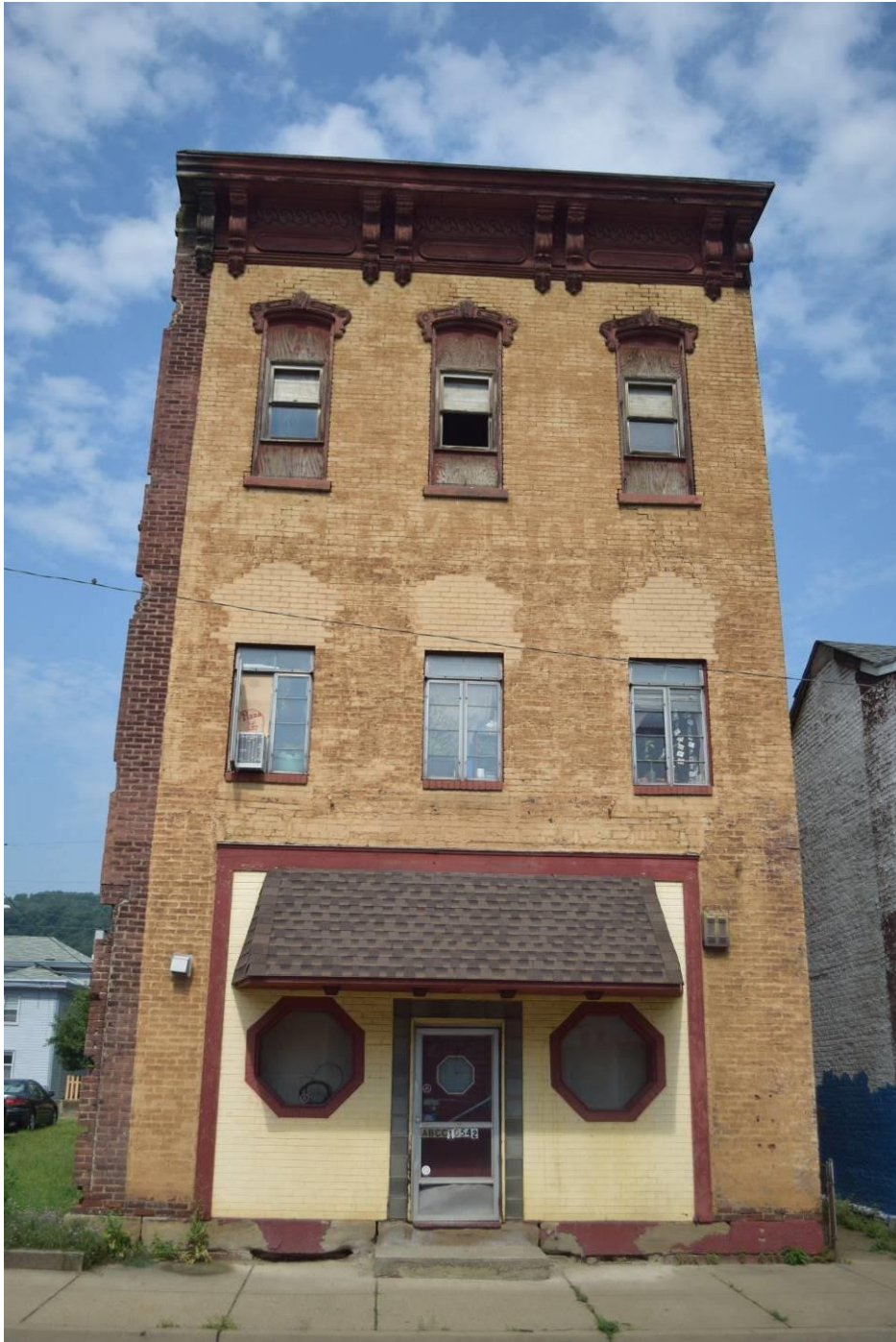
Photo 21. Three-story commercial building, 3719 Eoff Street, looking west. (R#190)
